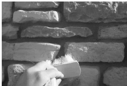
Final brushing of finished joints.
