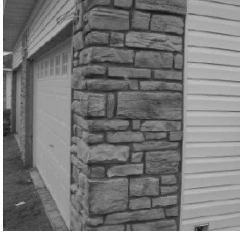
Alternate the long and short legs of corner pieces.
