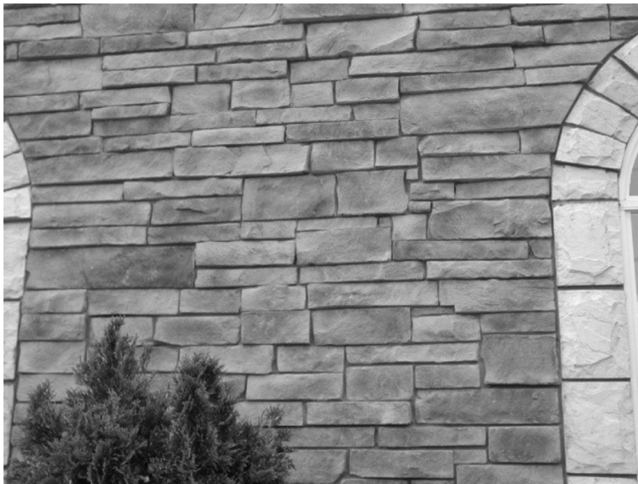
TriLite manufactured stone veneer installation example
