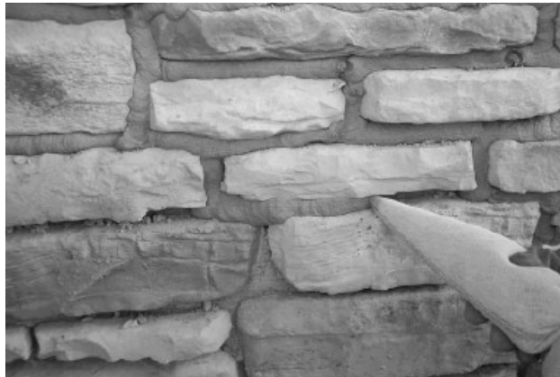
Tooling mortar joints after the mortar begins to firm.
