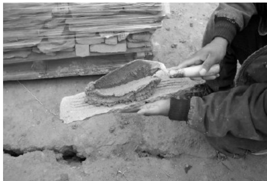
Applying setting mortar to the back of a veneer unit.
