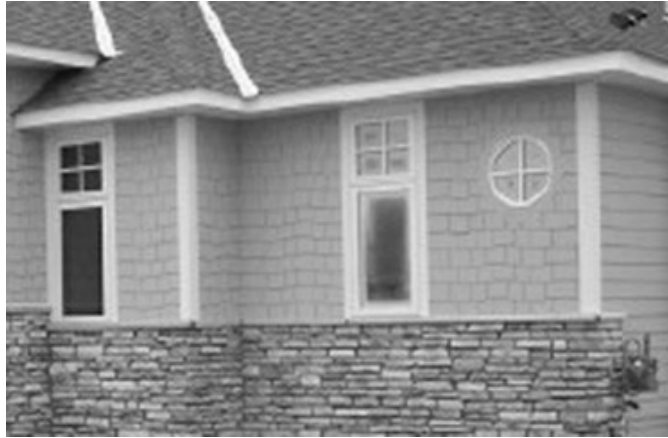
Project photo showing a finished sill/veneer condition.
