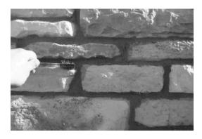
Perform the second step of finishing with a horse hair brush, which will gently remove lose mud and dust from the surface of the stone.
