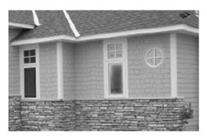
*TriLite Stone's Thin Brick:* The same instructions apply to installing TriLite Stone's Brick Veneer. However, extra care is needed to keep brick pieces level and consistently spaced. Snapping chalk lines is highly recommended to ensure consistency of lines.
