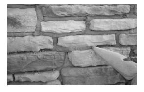
Grout is ready for the first step of finishing when it is scraped with a fingertip and crumbles, rather than smears. As grouting continues, it will be important to monitor the readiness of previously grouted areas. An effective finishing tool is a wooden lathe stick cut into 8" pieces. Scrape and compress top and bottom edge of each joint, knocking out any excess in the middle.
