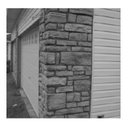
If application calls for grout joints, try to keep a consistent spacing between stones of 3/8", essentially the width of a thumb.
