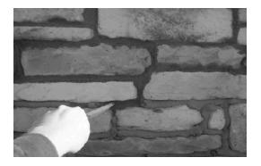
Smooth out the joints using a fine wire brush, checking for holes in the mud as you go. If holes are visible, use excess mud and fill them in with your fingertip.
