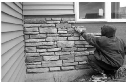
When installing flat stone, again, try to apply stone from top to bottom. However, Stackstone and/or Dry-stack styles may be easier to keep level if installed from the bottom up. In this case, be very attentive to mortar getting on the face of stones below.
