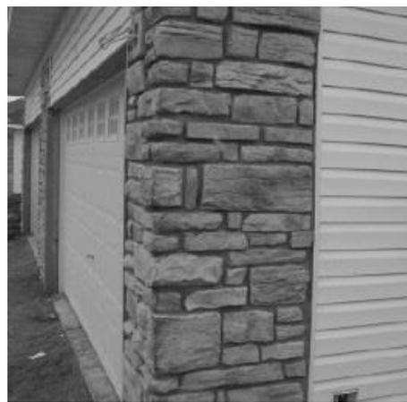
If application calls for grout joints, try to keep a consistent spacing between stones of  $\frac{3}{8}$ ", essentially the width of a thumb.
