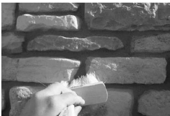
**Dry-stack (Mortarless) Applications:** Several of TriLite Stone's selections may be installed in a dry-stack fashion. These styles are produced to tightly fit together with little or no space between pieces of stone, meaning no grouting takes place.
